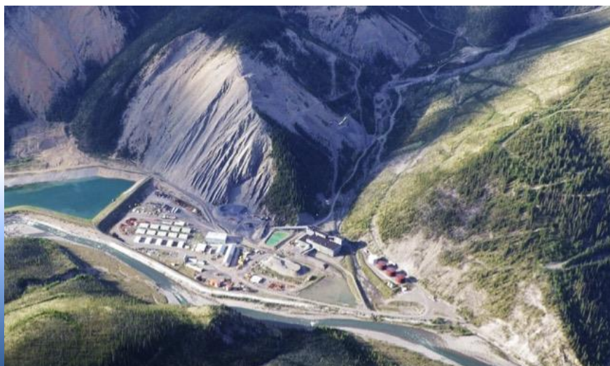
Canadian Zinc's Prairie Creek underground mine, which extends into the mountain behind the plant site in the photograph. (Photo: Canadian Zinc Corp.)
